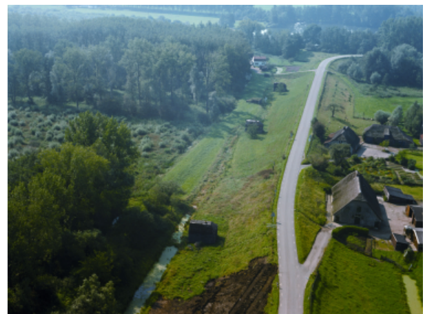
Photo 1 Historic compartmentalisation embankment (Diefdijk) which has been raised several times since it was first built in 1284.
