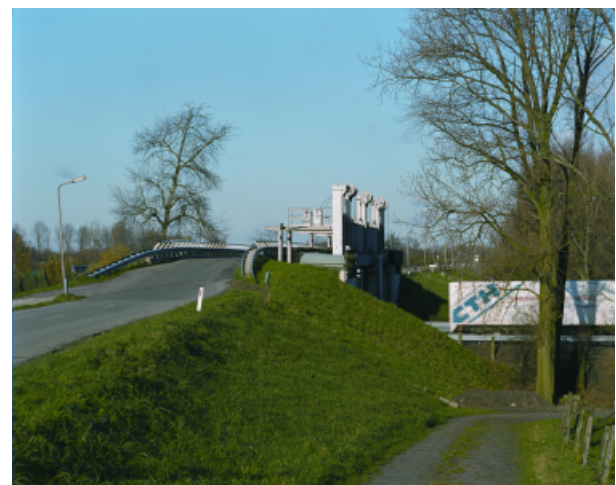
Photo 2 Cuts through compartmentalisation embankments should be avoided and it should at least be possible to close them in time (Diefdijk, 20th century situation). This issue was taken into account when assessing the robustness of various siting alternatives.
