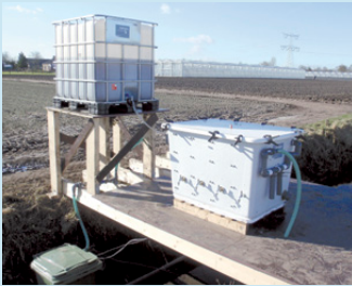
Field reactor for the removal of nitrate with ethanol injection in a ditch
