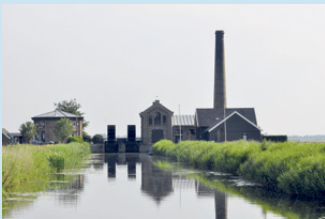
Historical pumping station
