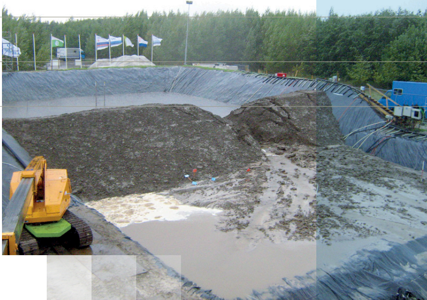
SBW Full scale piping experiment
