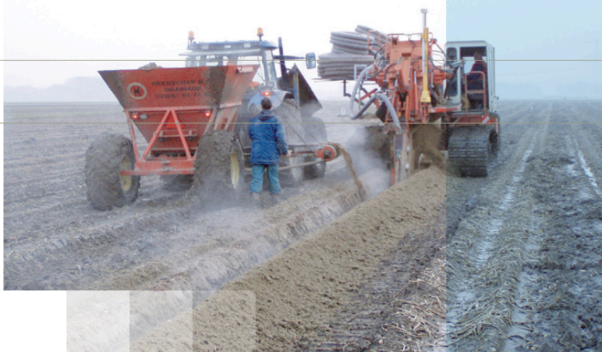
Installation of tile drainage with wood cuttings
