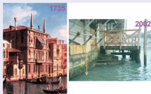
Figure 3. A view of Palazzo Christin-Lolin painted by Buffetti in 1735 (left), and a detail of the main entrance today (right). The algae skirt is 66 to 35 cm. The main staircase is now submerged and a new wooden wharf was necessary to enter.
