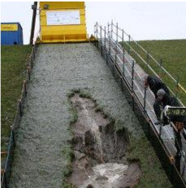
Figure 3.12 Failure of the inner slope of a levee as a result of a high overtopping discharge.
