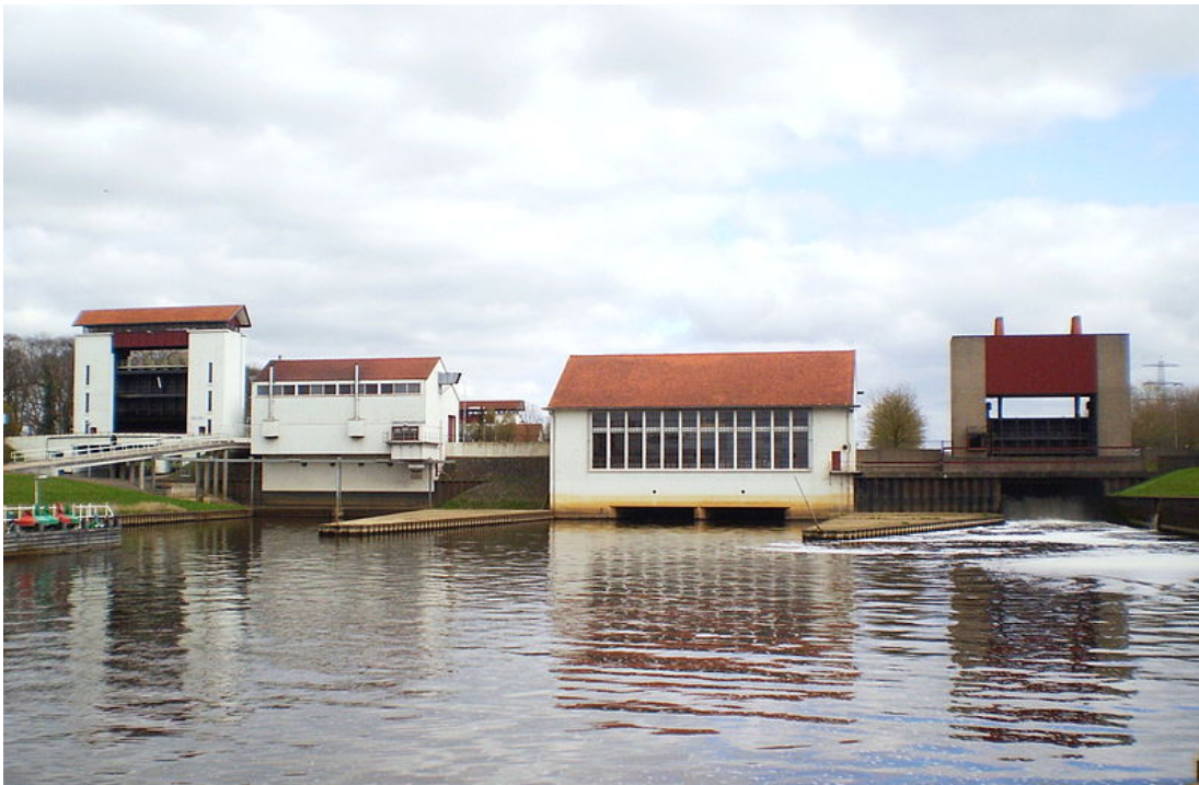
Figure 5.3: Sluice and pump complex "Eefde" in the Twenthe Canal near the IJssel river, the Netherlands (source: https://nl.wikipedia.org/wiki/Sluis_Eefde )
