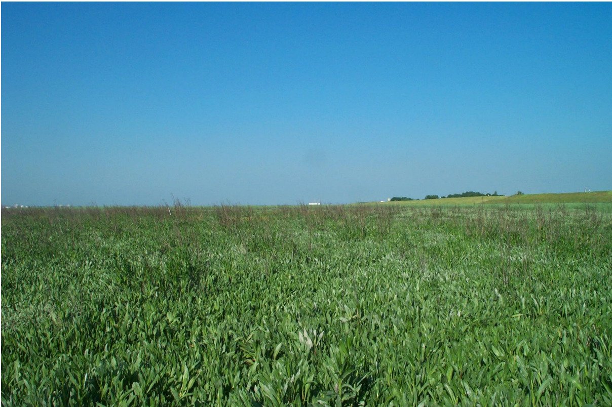
Saltmarsh vegetation providing protection against erosion of a dyke in the Netherlands. Photograph: Daphne van der Wal
