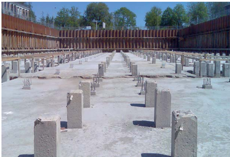
Figure 2 A typical Dutch deep excavation (Delft).
