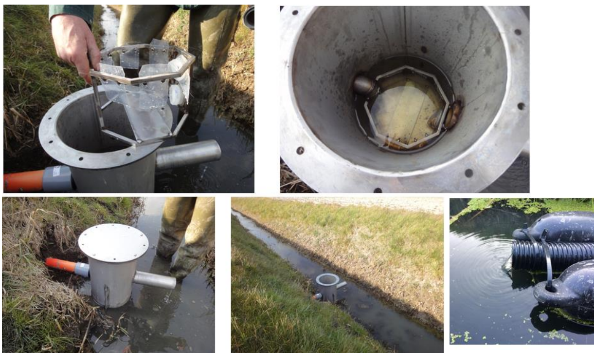
Figure 2.4 Installation of the samplers at the end of the drains
