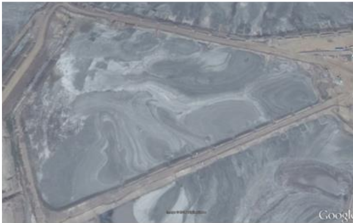
AFD and Tailings beaches
