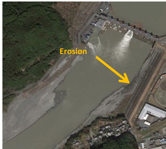
Figure 1. The erosion downstream of Funagira Dam (Source: Google-Earth).
