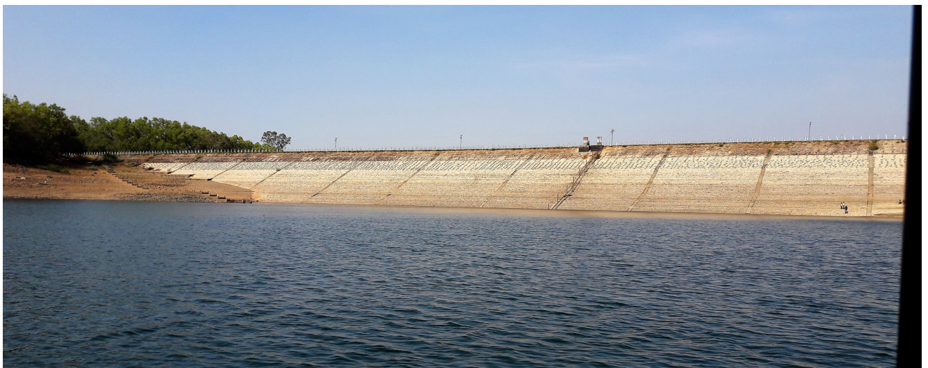
Figure 1 Bhadra embankment dam
