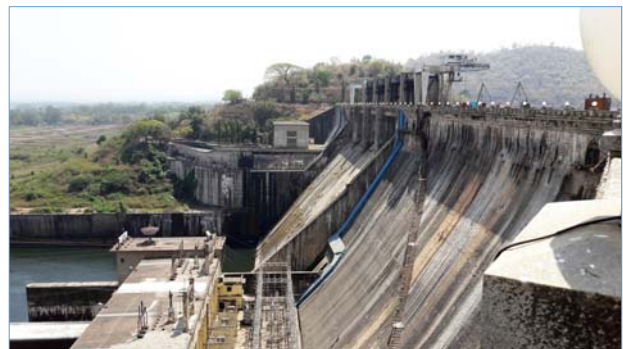
Bhadra dam (main dam)
