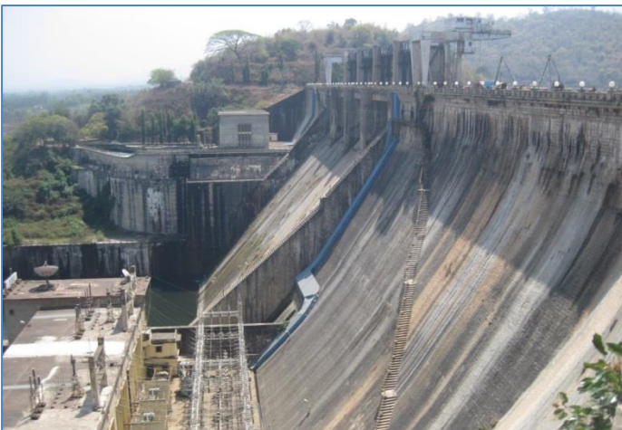
Fig.1 Masonry dam, Bhadra dam-reservoir system.
