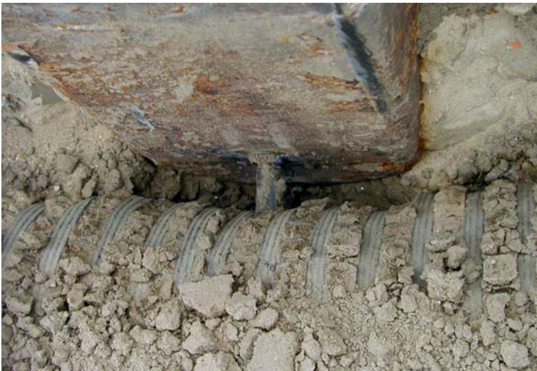
Foto 8 – Verbinding geogrid - damwand.
