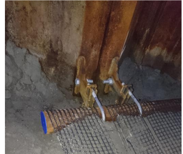
Geogrid anchoring of a sheetpile, Windpark Krammer WT17
