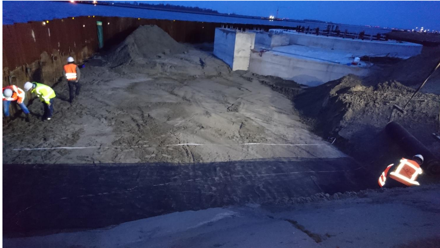
Looking in south direction from the embankment
