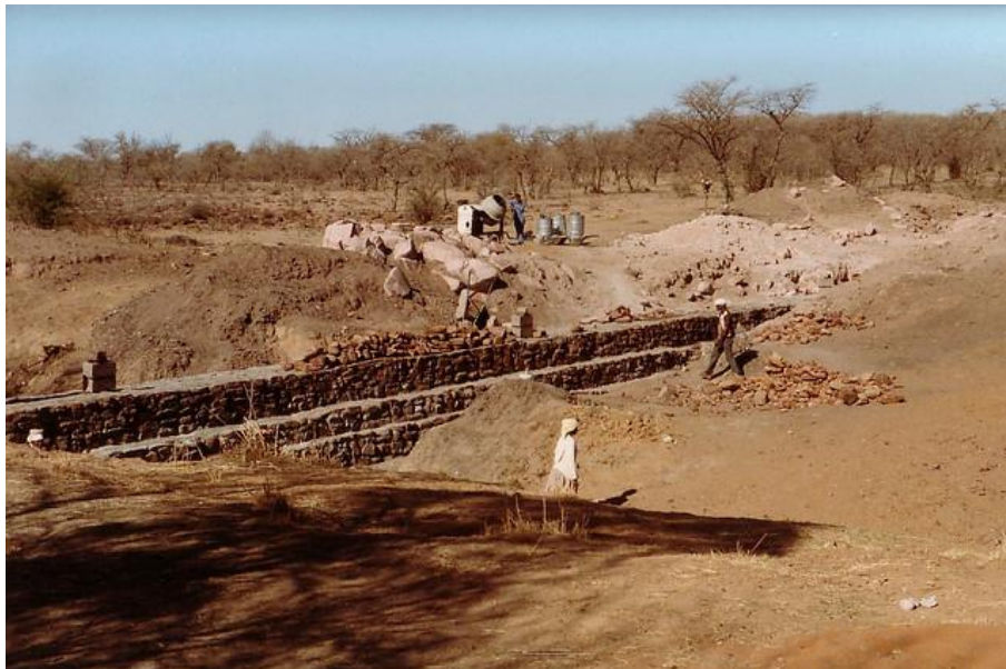
Figure 21: Weir construction in Botswana-labour intensive
