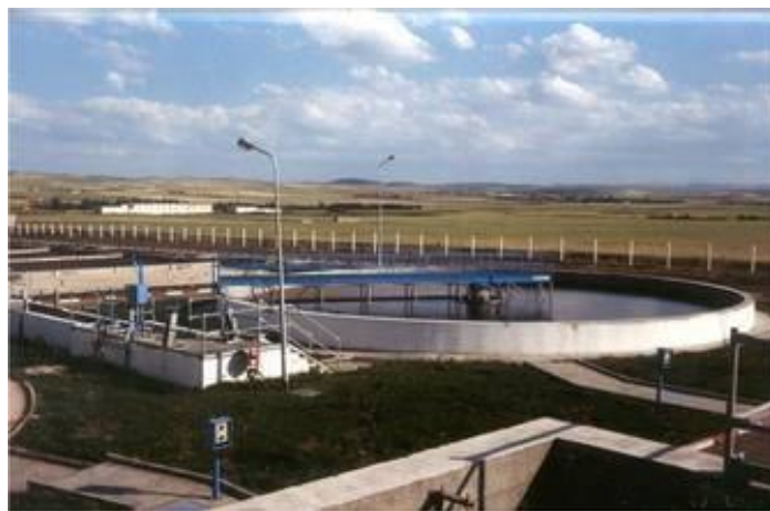
Figure 76: El kef waste water treatment plant in Tunis
