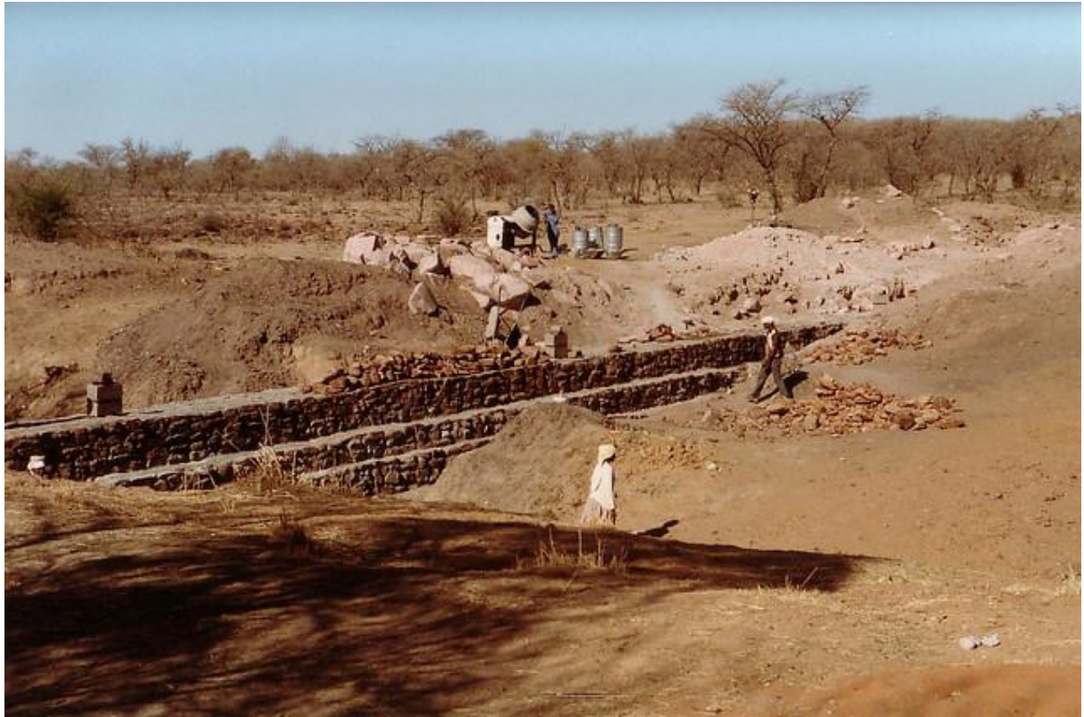
Figure 44: Weir construction in Botswana-labour intensive
