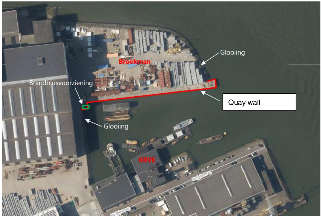
Figure 3.1 Position of the quay wall within the Sleepboothaven. The quay wall is indicated with the red line
