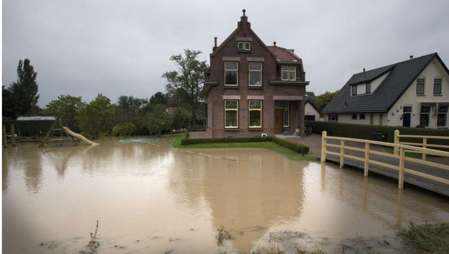
Figure 2: Flooding in the urban area of Stellendam. Retrieved from: Trouw, 2021
