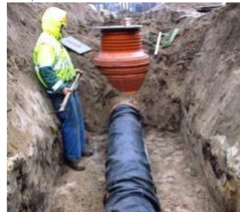
Figure 18: Infiltration transport pipe. (Source: Vergroesen et al., 2013)
