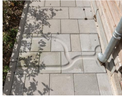
Figure 21: Rainwater tiles for controlled overland flow (Source: Struyk Verwo Infra, n.d.)
