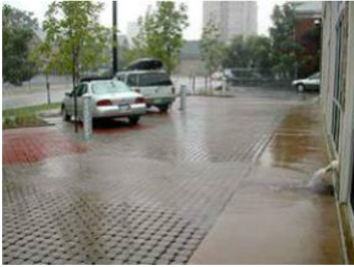
Figure 20: Permeable paved surface. (Source: Vergroesen et al., 2013)
