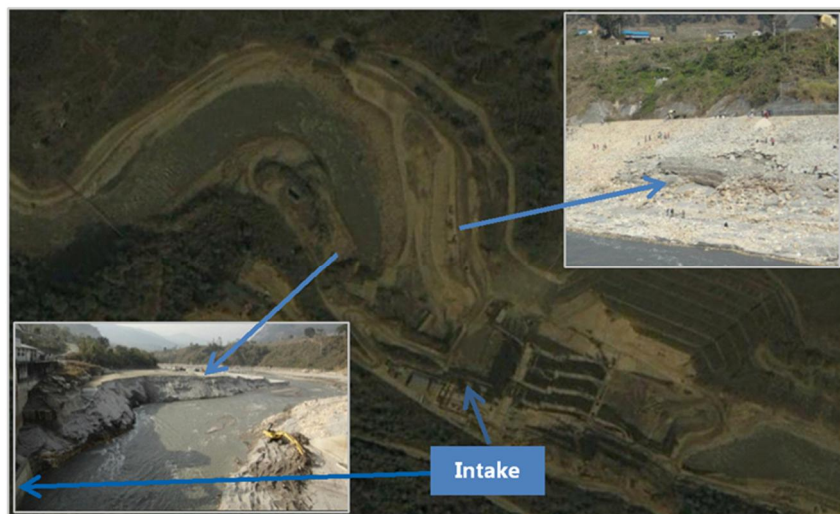
Figure 2. Sediment-induced problem at MMHEP (sedimentation at the inner bend and erosion at the toe of the outer bend) – The Google Earth image shows the reservoir condition of April 2008 (during construction), while the pictures were taken during drawdown for dredging and maintenance.
