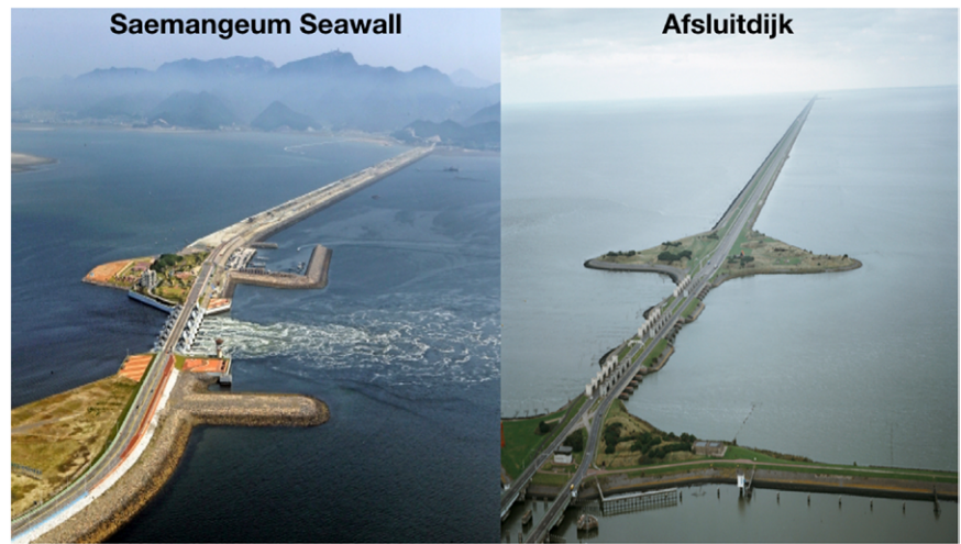
Fig. 2. Aerial views of (left) the Saemangeum Seawall in South Korea (source: https://structurae.net/en/photos/252428-saemangeum-seawall ) and (right) the Afsluitdijk in the Netherlands (source: https://beeldbank.rws.nl ), which are both over 30 km long.
