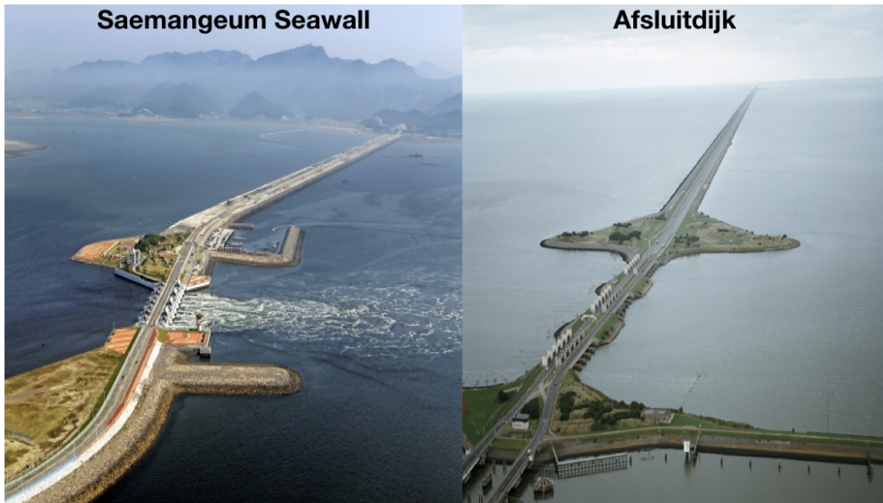
677 FIG. 2. Shown here are aerial views of the the Saemangeum Seawall in South Korea (Source: 678 https://structurae.net/en/photos/252428-saemangeum-seawall ) and the Afsluitdijk in the Netherlands (Source: 679 https://beeldbank.rws.nl ), which are both over 30 km long.
