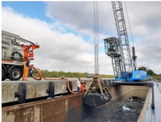
(c) Pumping the mud from the hopper into the truck for transport to Deltares.
