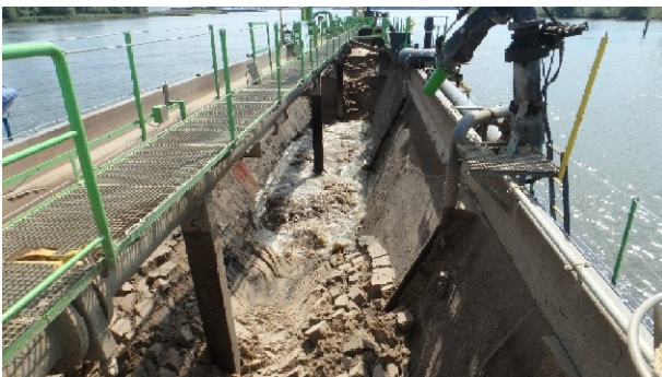
Figure 1. Nourishment operation, unloading above a deep scour hole in the ‘Oude Maas’ River, June 2022
