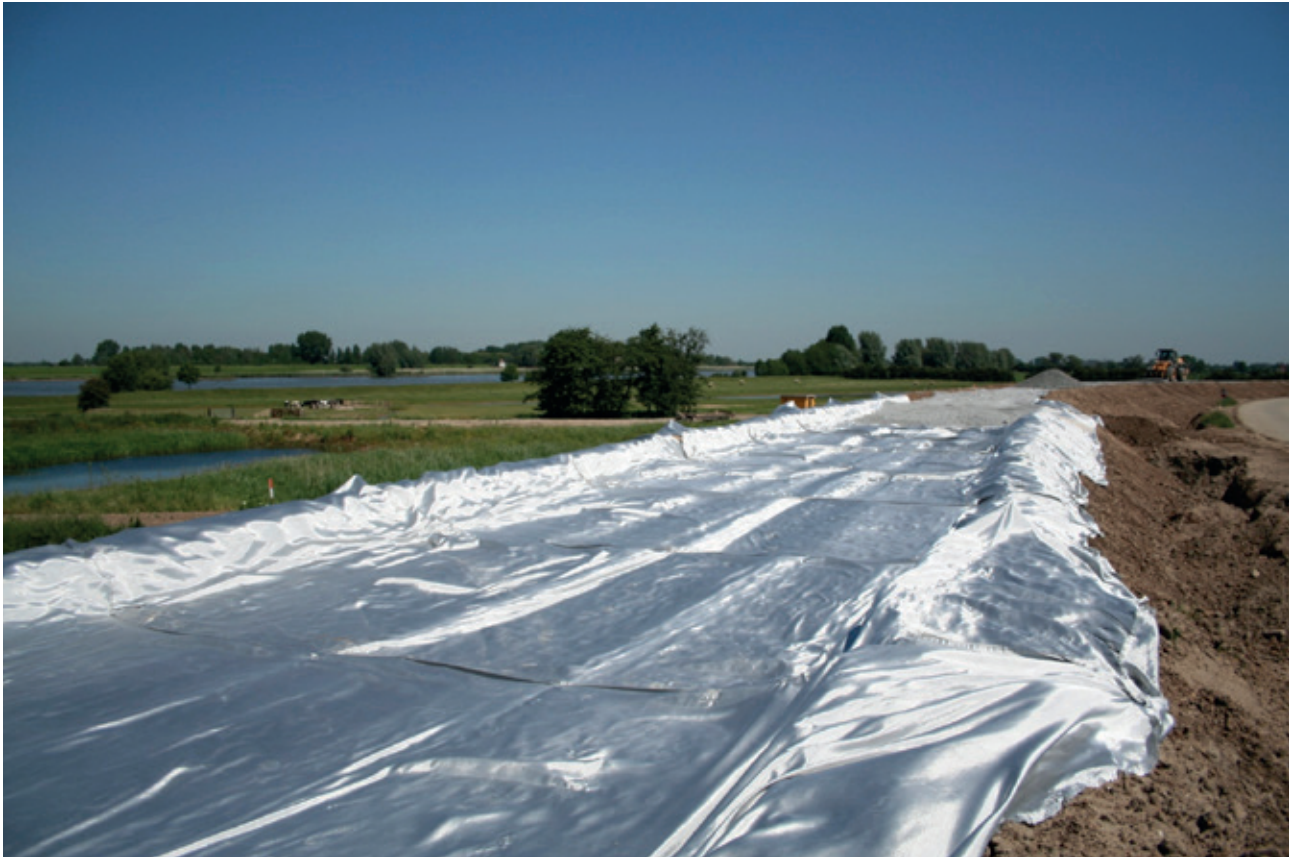
Foto: Project dijkverbetering Hagestein-Zederik (C. Brok, 2006)
