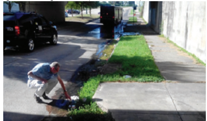
Measuring salt seepage at Press Drive (below railroad bridge)
