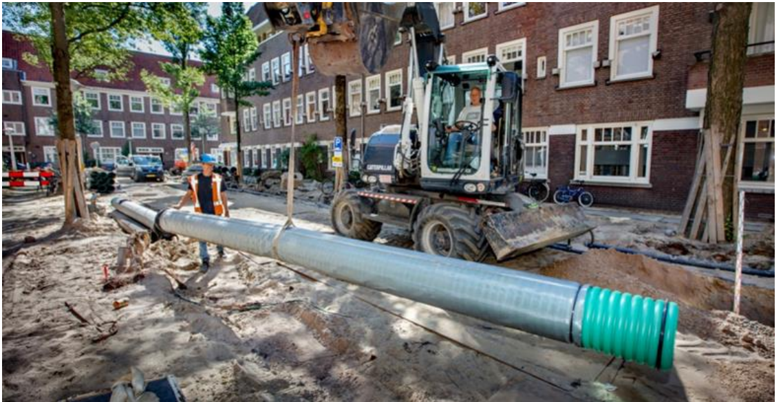
Figure 5.5: Installation IT-drain in Amsterdam (Amsterdam Rainproof)
