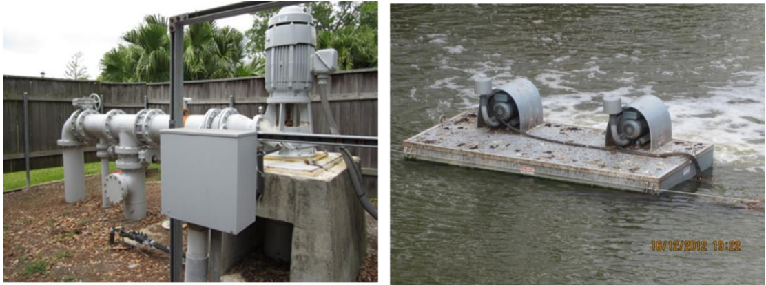
Figure 3.10: Groundwater pump and machines adding air into the ponds.
