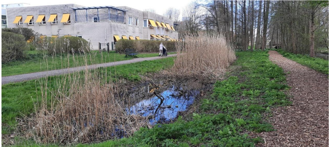
Figure 5.6: An example of a simple and cheap vegetated storage pond (constructed wetland) in Amstelveen (the Netherlands). Maintenance: mowing reeds once a year. Construction: digging a depression connected with parking of local hospital.
