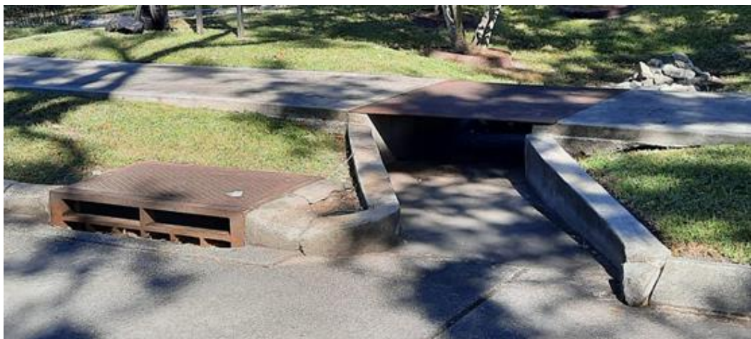
Figure 7.1: Example of a catch basin next to bioswale inlet.
