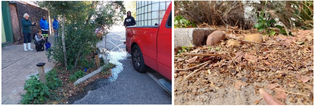
Figure 6.14 Water cannot enter the rain garden (blocked or to drain next to inlet rain garden)
