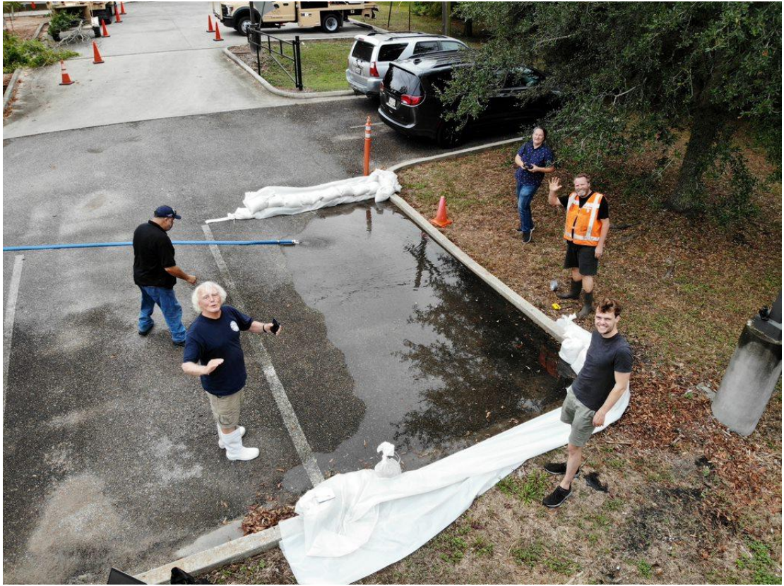
Full scale testing of permeable pavement (City Park, picture Ramiro Diaz).
