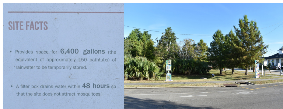
Figure 4. (Left) Sign at green infrastructure site ‘drains water within 48 h so the site does not attract mosquitoes’ source: https://www.climatescan.nl/projects/7399/detail , accessed on 20 December 2022. (Right) Test location with signs on the right of the inlet.
