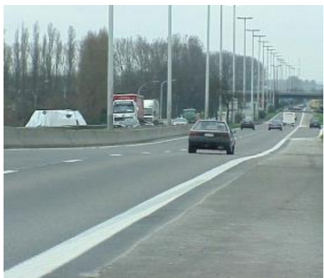
Figure 5.1.1: Undulating road. Source: (Charlier et al., 2018)
