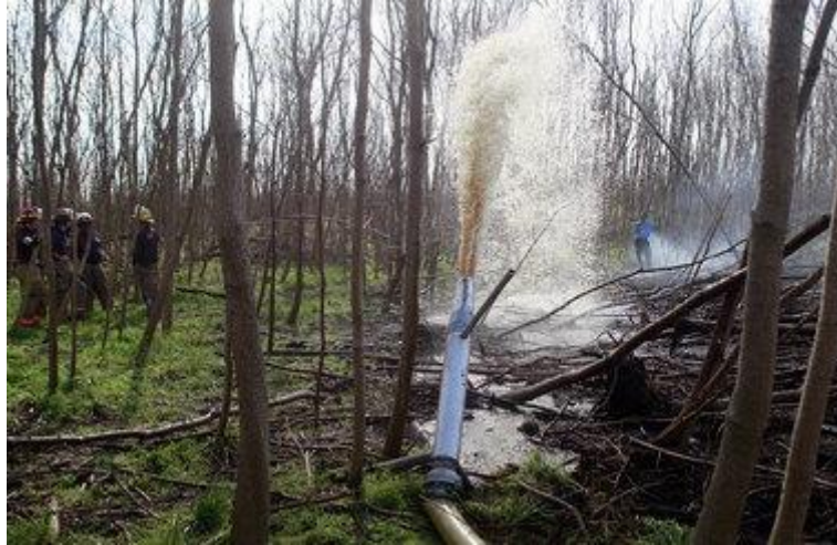
Figure 6.3.6: David Grunfeld, The Times-Picayune The New Orleans Fire Department fights the underground fire in eastern New Orleans on Jan. 17 by pumping water from a nearby canal to the site using a 6-inch fire hose. Source: (Schleifstein, 2012)
