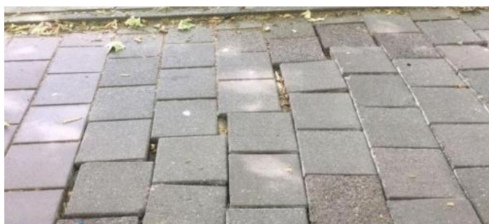
Figure 5.1.3: Loose tiles due to dehydrated soils in Haarlem. Source: (Haarlems Weekblad, 2018)
