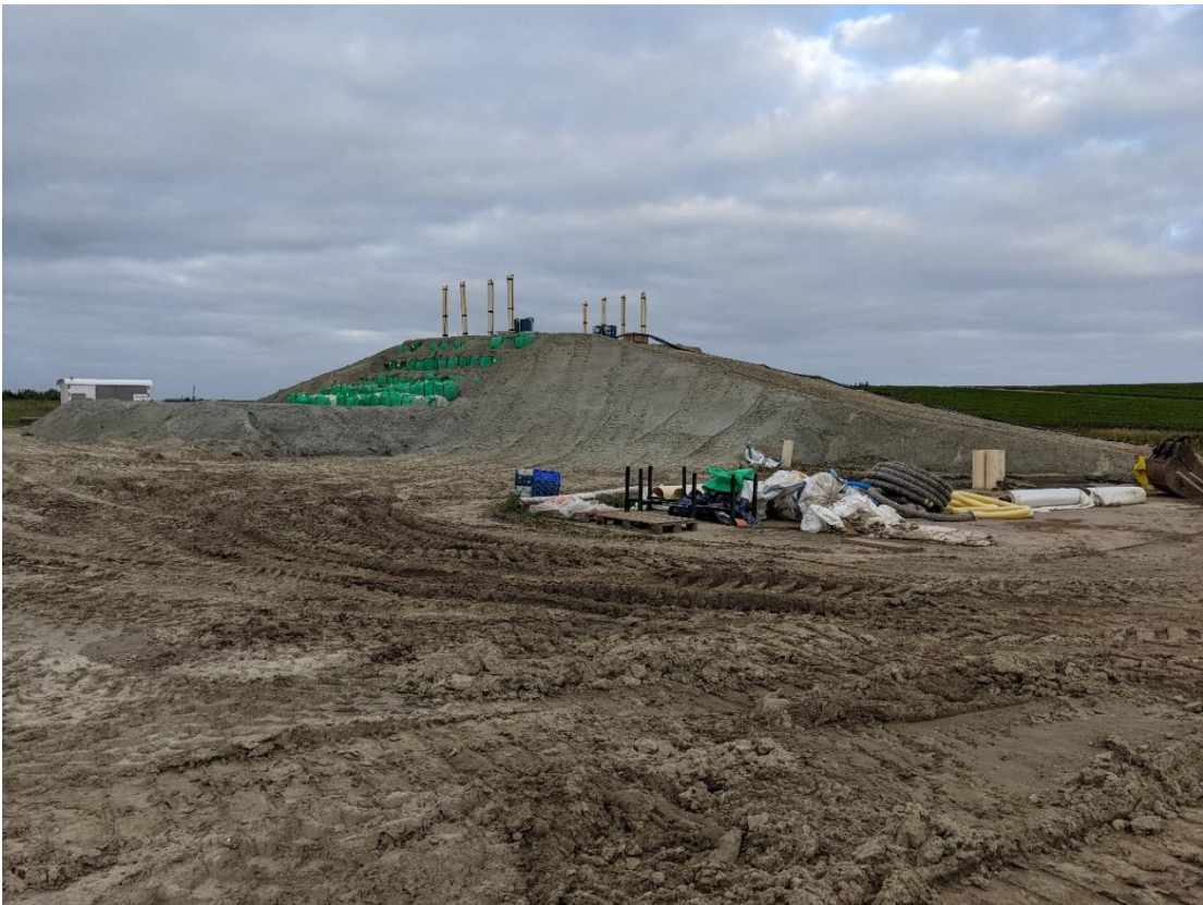
Figure 2 The constructed levee
