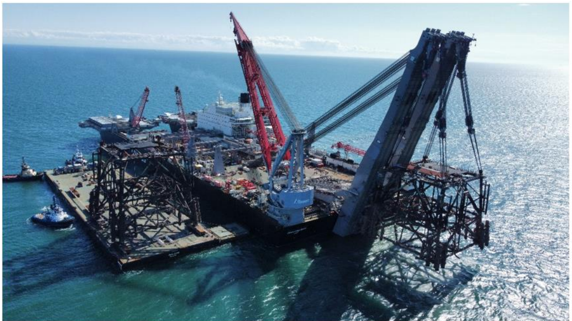
Figure 6.1 Allseas Morecambe project. The Pioneering Spirit lifting the second offshore jacket with Iron Lady moored next to it. Operations are timed favourably (during slack water) by means of the TKI Ocean Race Pilot.
