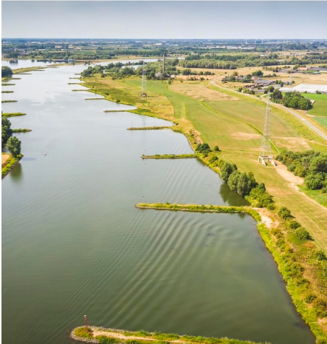
The river Nederrijn in between Wageningen and Rhene, with the Grebbedijk visible on the right (WSP Global)
