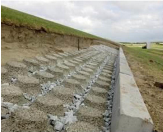
Figuur 5.3. A revetment consisting of two layers
