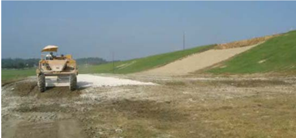
Figuur 1: Preliminary mixing of lime and embankment soils in mixing area
