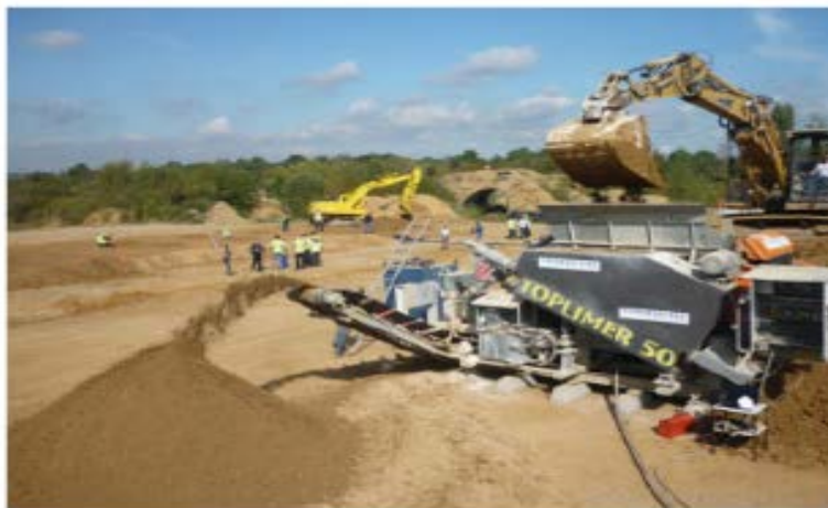
Figure 1. Lime-treated material production with a mixing and treatment mobile plant.
