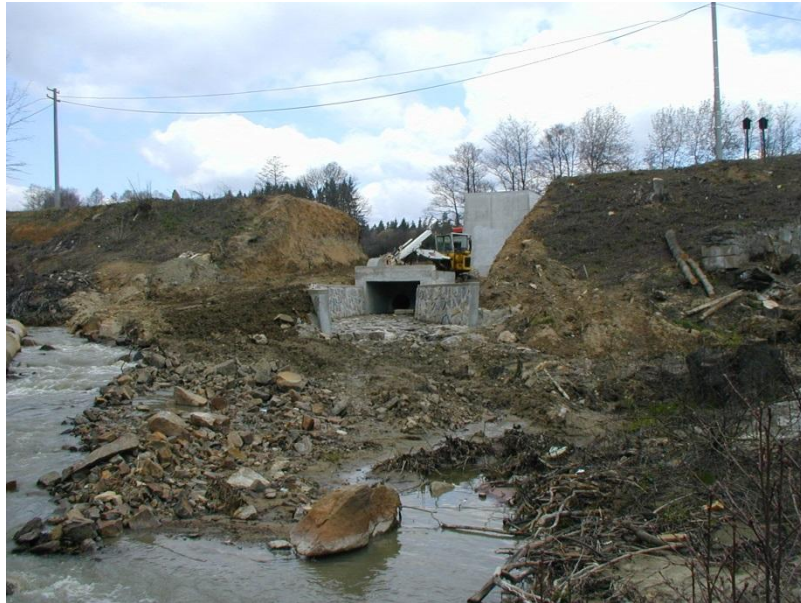
Figure 3.5. Destroyed dike of Chobot pond near Milevsko during floods in 2002.
