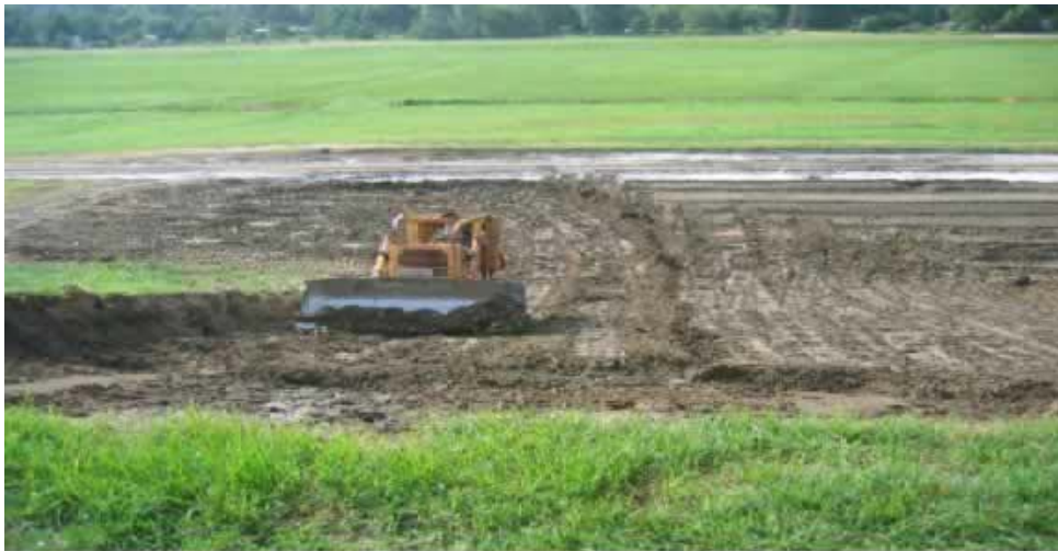
Figure 2: Returning treated soils from mixing area to embankment
