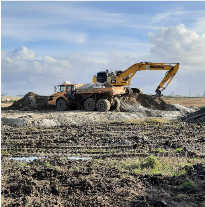
Figure 3-10 Excavator and transport truck on the production platform.
