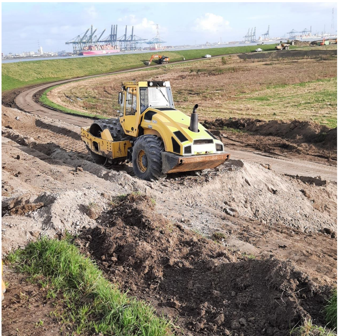
Figure 3-7 Densification in horizontal layers in the Hedwigepolder.
