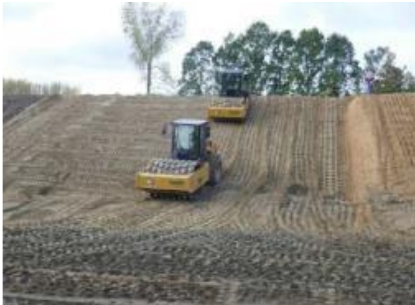
Figure 3-5 Compaction of the treated soil along the slope (Vlassenbroekpolder).
