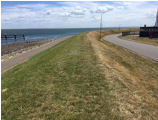
Figure 13. Shadow side (left) sunlit side (right) of a levee in Yerseke (van Grinsven, 2020).
