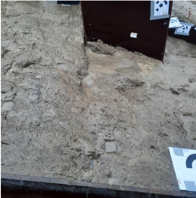
Figure 8-8 Shortly before the construction failed; the erosion has deepened to a maximum of (locally) 50 centimetres.
