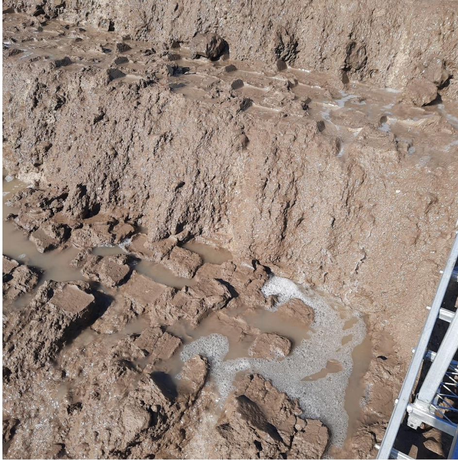
Figure 8-3 Footprint of the compacting machine.
