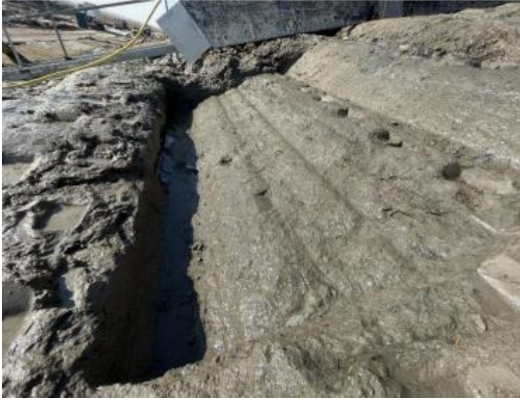
Figure 6-12 Situation after the final test (picture courtesy of Infram).
