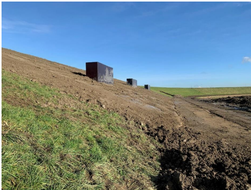
Figure 3-9 Side view of completed test sections.
