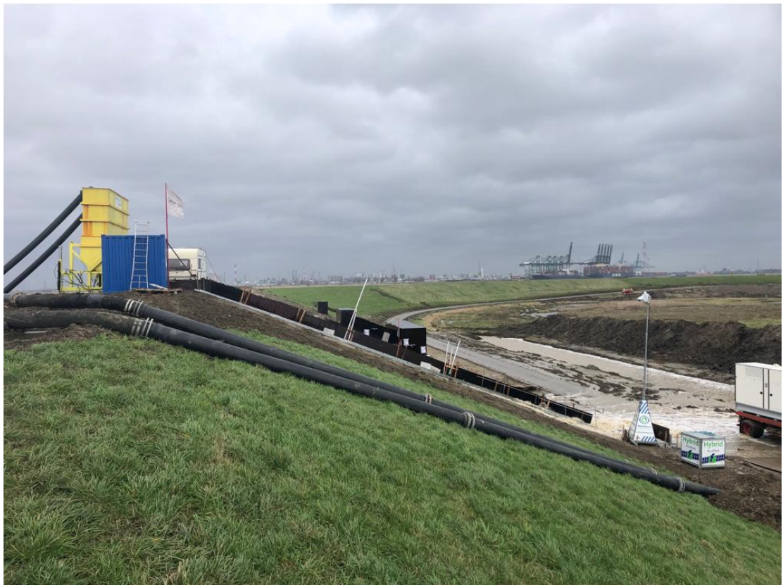
Figure 5-1 The wave overtopping simulator (WOS) on site at the Hedwigepolder.
