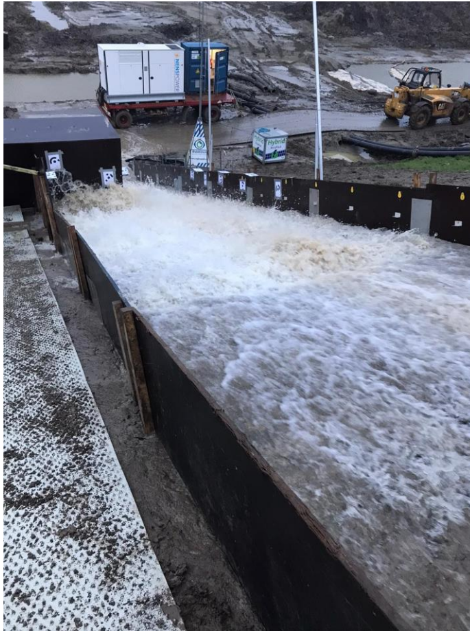
Figure 5-4 The wave overtopping simulator at work.
