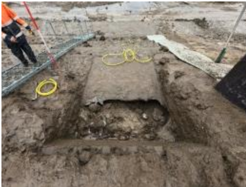
Figure 6-10 One step has been eroded and the next step is seriously undermined (picture courtesy of Infram).
