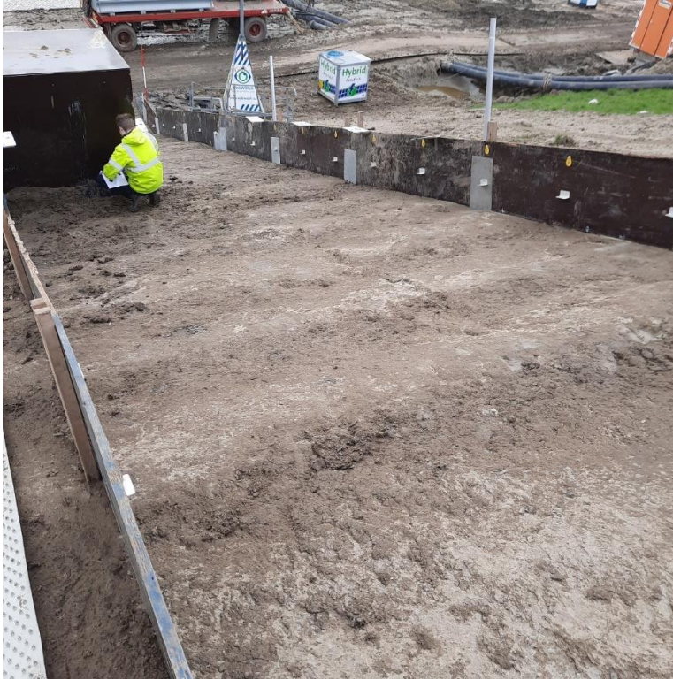
Figure 8-1 Situation in Section 1A before the start of the overtopping tests.
