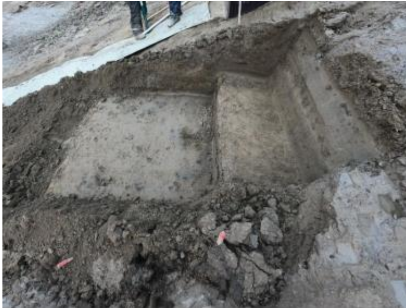
Figure 6-9 The situation at the start of the extra test: the original stair case is exposed to wave action (picture courtesy of Infram).
