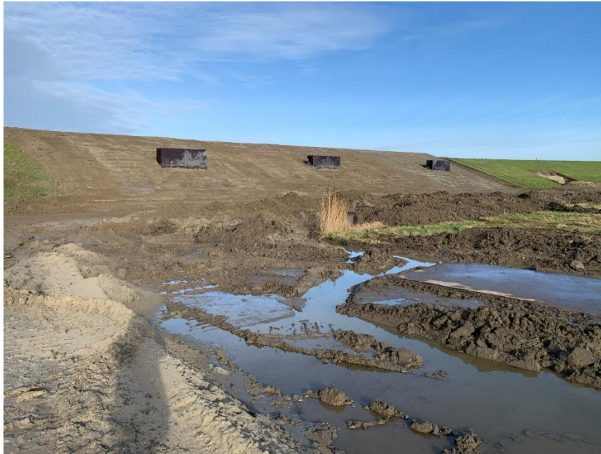
Figure 3-8 Completed test sections with objects. From left to right: Section 1 with Poor quality clay A, Section 2 with Poor quality clay B and Section 3 with Good quality clay.
