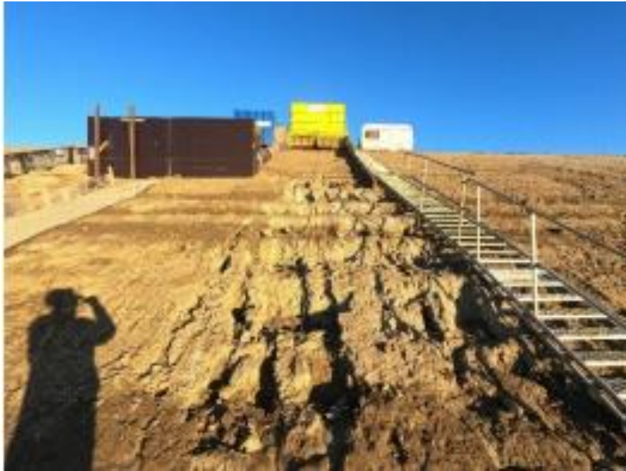
Figure 6-8 Before the start of testing in section 2B.
