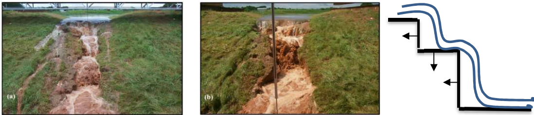
Figure 2: Headcut erosion processes during overflow (After Hanson, 2005)
