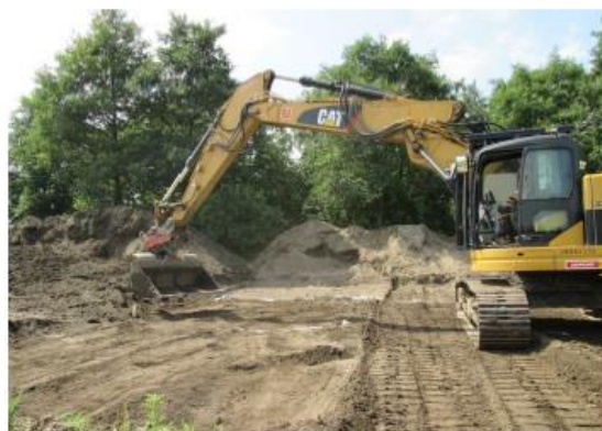
Figure All.135. Compaction with the excavator shovel only
