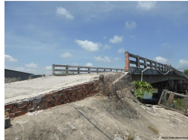
Shallow subsidence, visible around founded bridges and buildings
