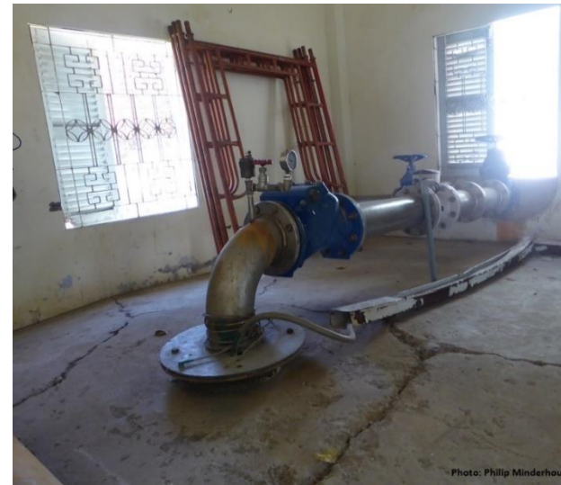
Deeper subsidence, visible by protruding pumping wells
