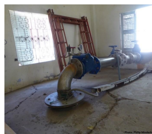
Deeper subsidence, visible by protruding pumping wells
