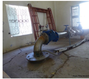
Deeper subsidence, visible by protruding pumping wells
