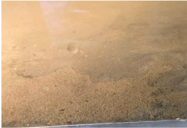
Figure B. 9: Development of surface erosion for Test BA-APP.
