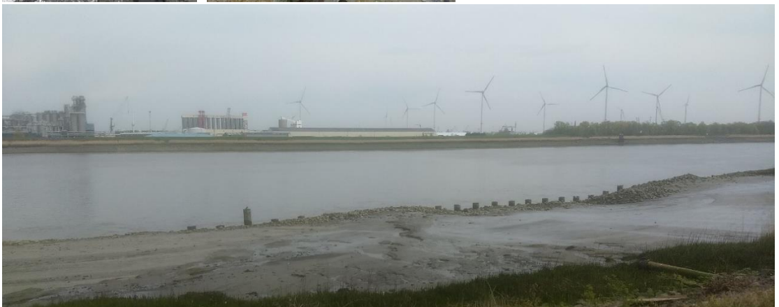
Figure 6-32: Sampling location Oosterweel near Antwerp. Loc 1: At the low water level line; Loc 2: Low water level line +8 m towards the shore; Loc 3: Low water level line +24 m towards the shore
