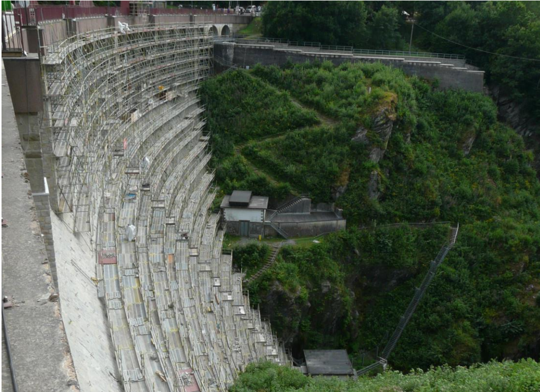
The dam (under revision)
