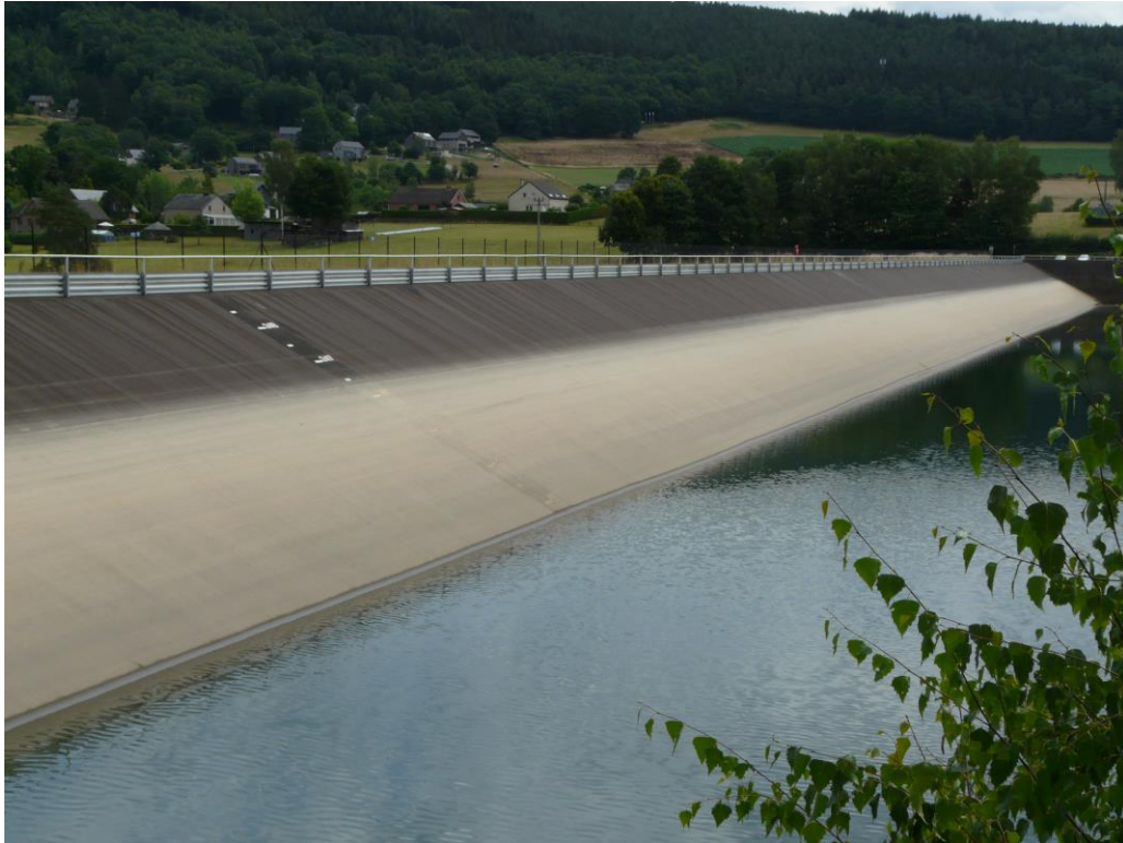
Lower basin of pumped storage plant
