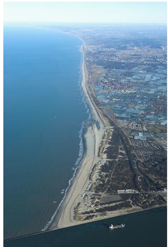
Figure 1.1 Overview project site
