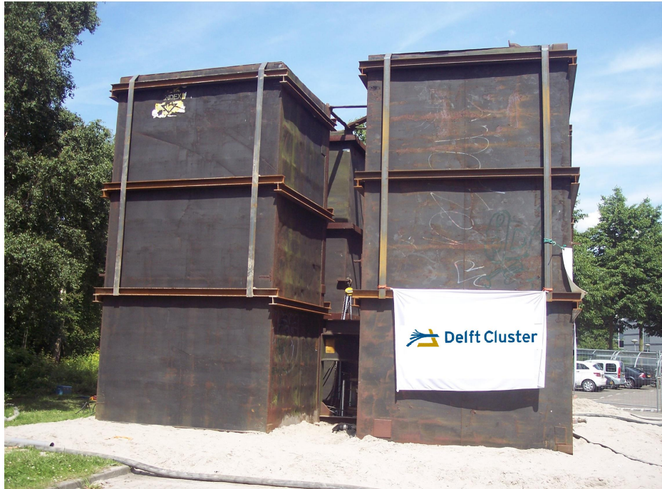
Static Load Testing load step 1 hour (full test 1 day) weight 100% (of capacity)
