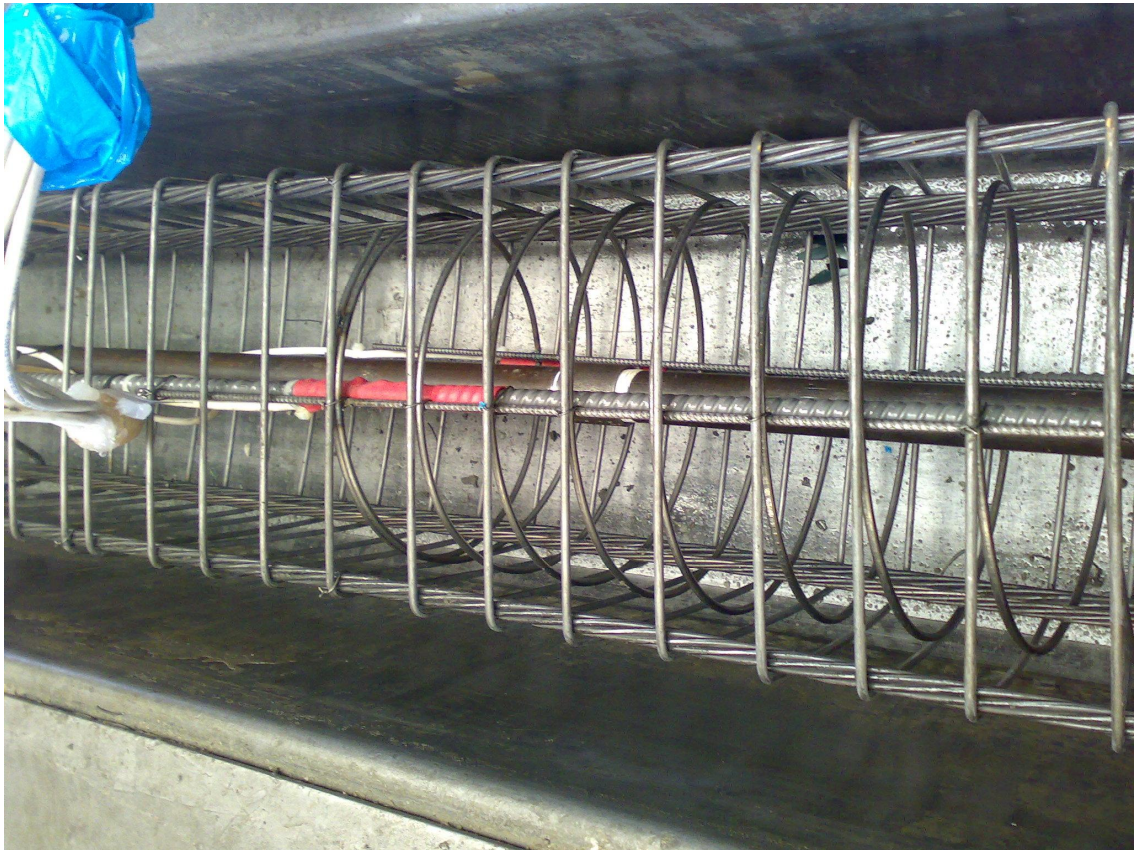
Photo 3.1 Strain bar and reinforcement of the pile
