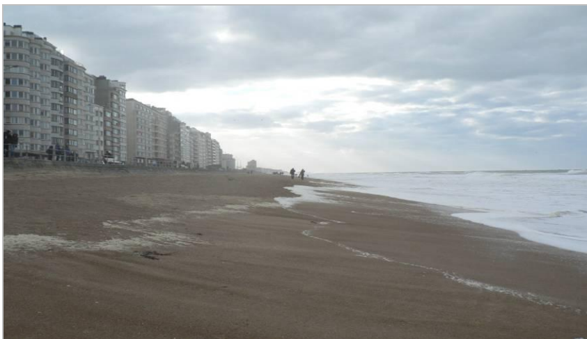
Figure 6.8 Dyke and beach at Ostend centrum.
