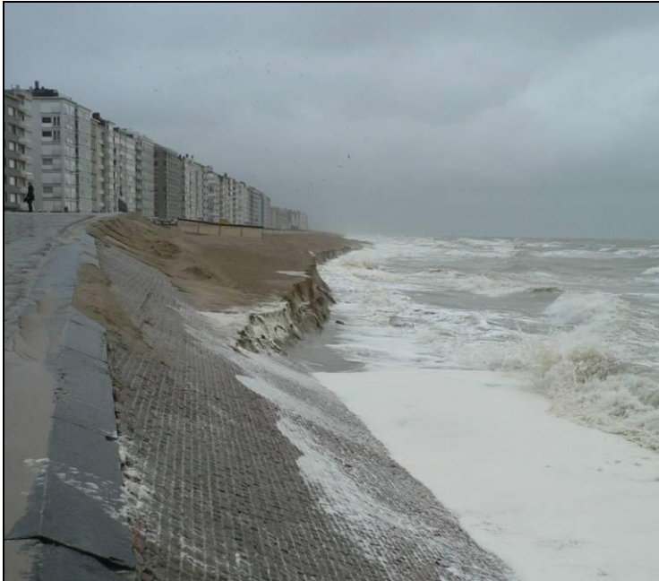
Figure 6.7 Beach scarp erosion (storm with 1/10 yr return period)
