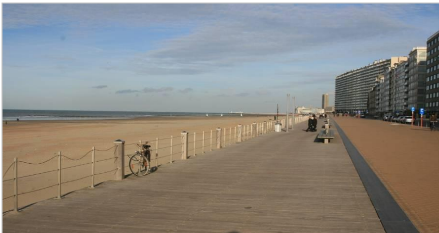
Figure 6.4 Dyke, promenade and beach at Mariakerke. Note the apartment buildings on the dyke
