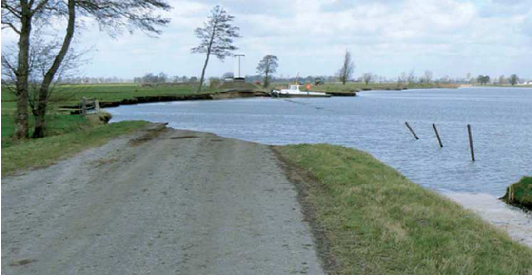
Figure 2.2-1: Result of a breach flow slide (2008).
